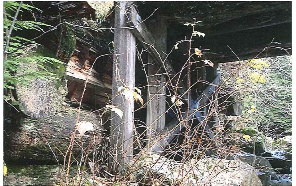
CK2176 Abutment Right Bank
