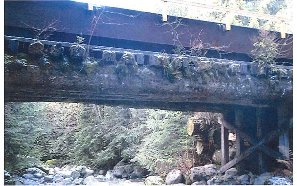
CK2176 Crossing upstream
