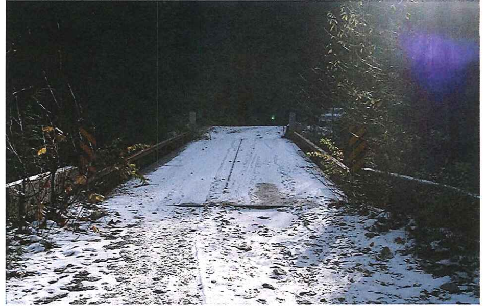
CK2176 Approach Right Bank
