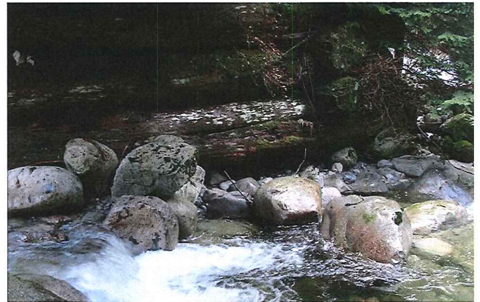
CK2176 Abutment Left Bank
